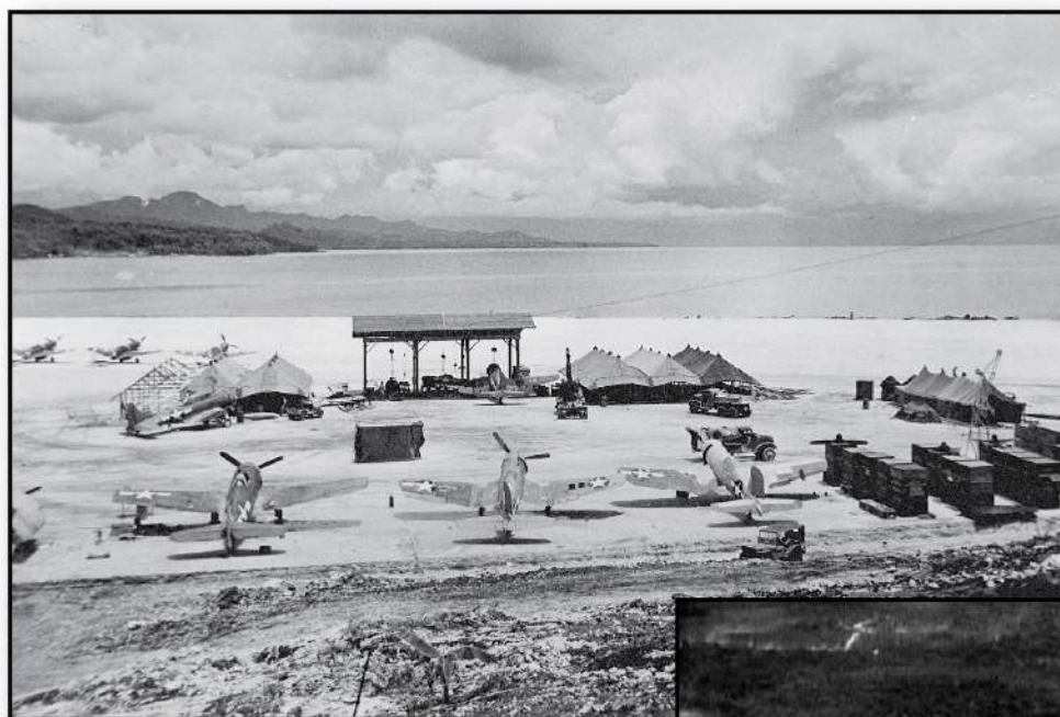
At left is an atmospheric shot of Vella Lavella airfield from December of 1943. Visible are Corsairs, Hellcats, a wingless SBD, and out near the beach a trio of RNZAF Kittyhawks. The tents house various maintenance shops, with a more permanent structure with hoists for prop and engine changes.
