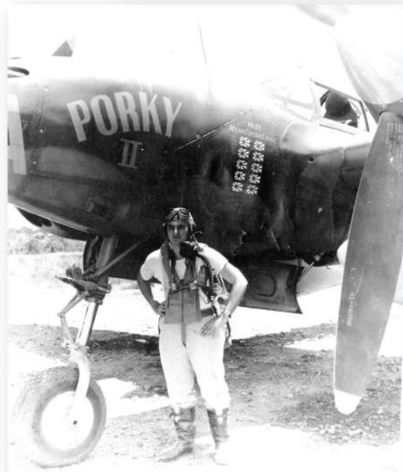
"Porky II" showing her covered nose, and uncovered main wheel hubs. Again, note the light grey Mk.6 tanks - noticeably lighter than the Neutral Gray belly of the aircraft. Cragg's ship appears to be fairly well maintained (given the conditions...). Note the ubiquitous light brownish grey exhaust and tetraethyl lead stains on the boom and the vertical fin.
