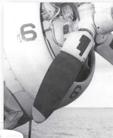
Above: Front view of prop showing white area out to the edge of the cowling. Many times the blade data block on the cuff, and sometimes the blades above the cuff were masked off. Back sides of blades were not painted. In the photo, note how the white covered visible parts of the engine, including the reduction gear housing, magnetos, ignition harness, and even the cylinders themselves.
