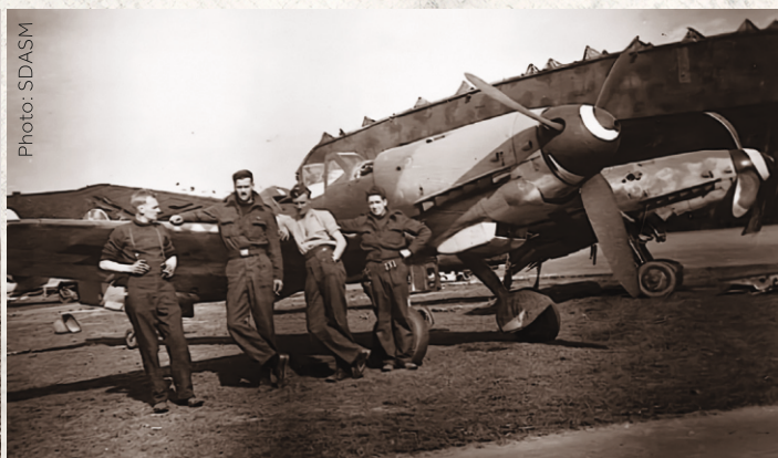
Photo: SDASM Allied soldiers in Wunstorf in second half of 1945 in front of Bf 109 K-4 WNr. 332 700. The machine shows late style camouflage and simplified crosses on lower surfaces of the wing. In the background is visible WNr. 330 255 "Black chevron" of Stab III./JG 27 with early style camouflage and black/white crosses on lower surfaces.
